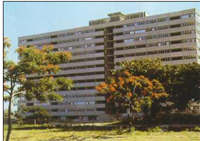
Precast Prestressed Concrete Frame with Concrete Shear Walls
